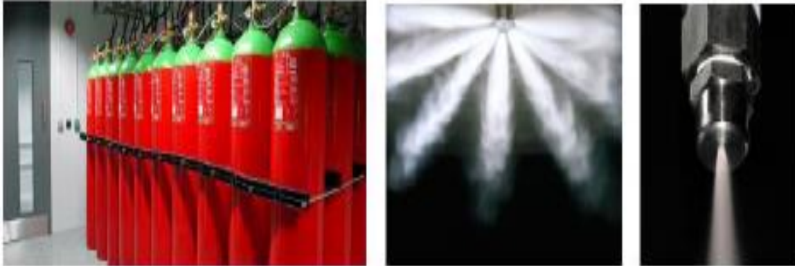
Figure 28: Clean agent systems
